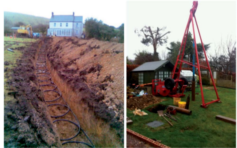
Fig. 6 The installation of ground loops for GSHP systems using slinky horizontal pipes (left) and a vertical borehole (right). source: Staffell et al, 2012
