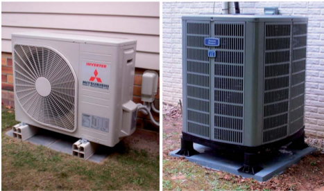
Fig. 5 Examples of air source heat pumps from Mitsubishi (left) and American Standard (right).
